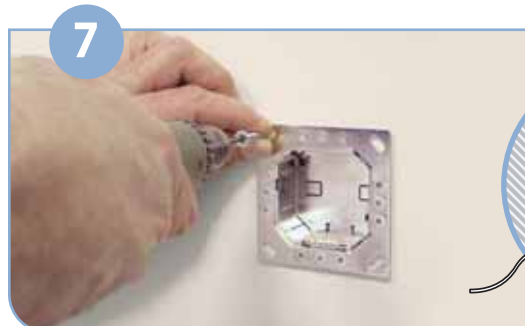
Make sure that the Housing is fully inserted, level-headed and Housing contacts are located at the bottom part as shown in picture. Secure with 4 screws.
