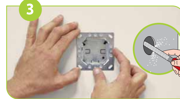
Trim the cutout gently and check that the Housing fits in properly.
