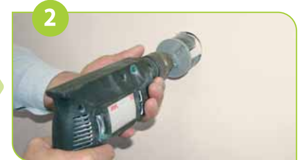
Drill the wall cut out at the designated location. Warning! Make sure not to drill next to electricity / telephone lines. Test for existence of power lines or enforcement beams prior to drilling the wall cutout.
