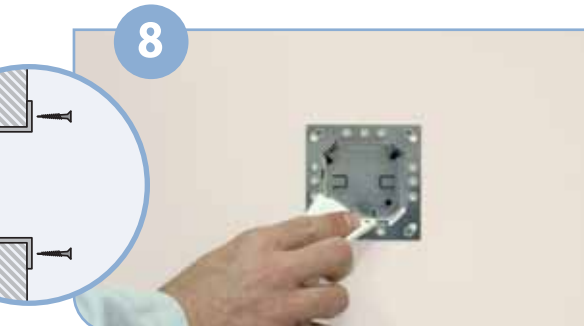
Gently clean the Housing contacts from dust and other objects.
