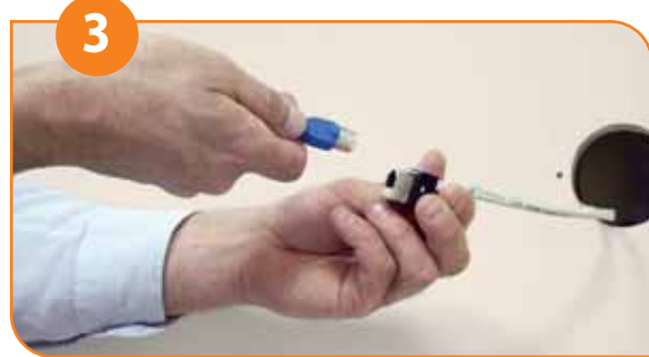
Pull out the LAN cable. Take the RJ-45 Termination Connector Block, which is not supplied in default packaging and needs to be purchased separately.
