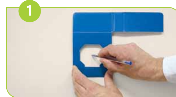
Use the lower Cardboard template supplied in packaging to mark the designated wall cutout for the Housing installation.
