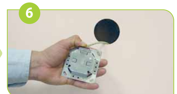
Close the IDC Krone Termination Connector Block and insert it into the Housing bottom part until you hear a clicking sound indicating it has locked properly into place.
