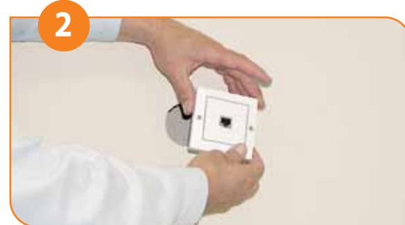
Remove the existing LAN Jack from the wall. Separate the LAN Jack module from the front panel.
