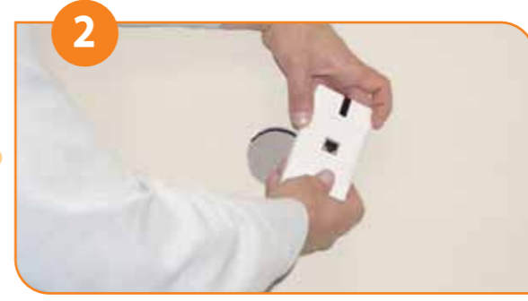
Remove the existing LAN Jack from the wall. Separate the LAN Jack module from the front panel.
