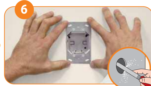
Place Housing inside the wall cutout. Trim wall cutout if necessary.
