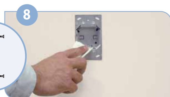
Gently clean the Housing contacts from dust and other objects.
