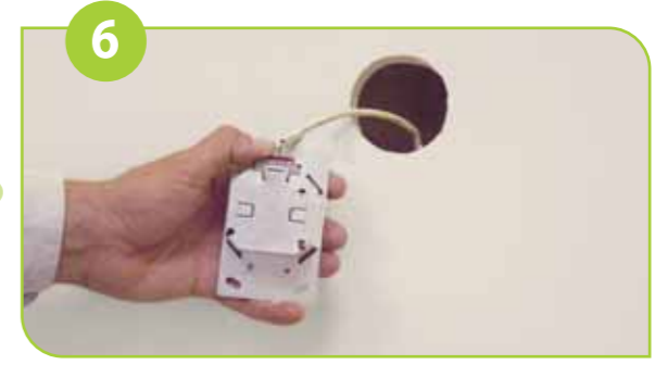
Close the IDC Krone Termination Connector Block and insert it into the Housing bottom part until you hear a clicking sound indicating it has locked properly into place.
