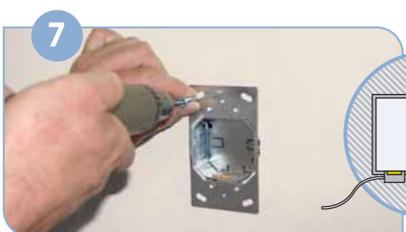
Make sure that the Housing is fully inserted, level-headed and Housing contacts are located at the bottom part as shown in picture. Secure with 4 screws.
