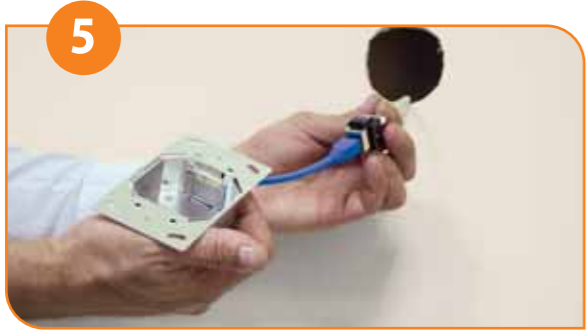
Insert the RJ-45 Termination Connector Block into the Housing bottom part until you hear a clicking sound indicating it has locked properly into place.
