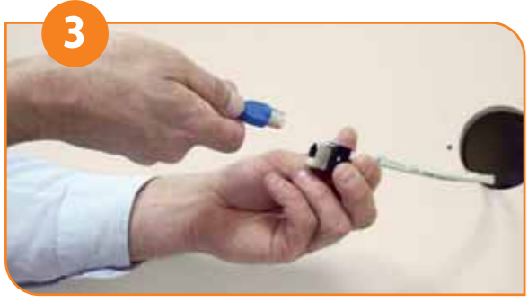
Pull out the LAN cable. Take the RJ-45 Termination Connector Block, which is not supplied in default packaging and needs to be purchased separately.
