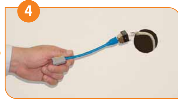
Connect the LAN jack and RJ-45 connector on the RJ-45 Termination Connector Block.
