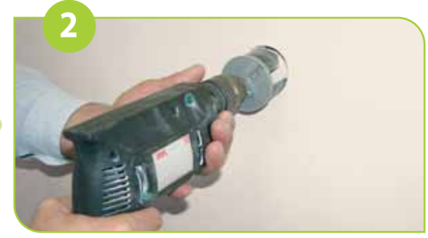
Drill the wall cut out at the designated location. Warning! Make sure not to drill next to electricity / telephone lines. Test for existence of power lines or enforcement beams prior to drilling the wall cutout.
