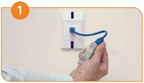
Use Power-over-Ethernet tester to check existence of PoE in the Jack designated for installation.
