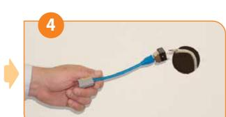
Remove the existing LAN Jack from the wall. Separate the LAN Jack module
