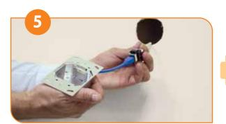
Insert the RJ-45 Termination Connector Block into the Housing bottom part until you hear a clicking sound indicating it has locked properly
