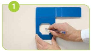
Use the lower Cardboard template supplied in packaging to mark the designated wall cutout for the Housing installation.
